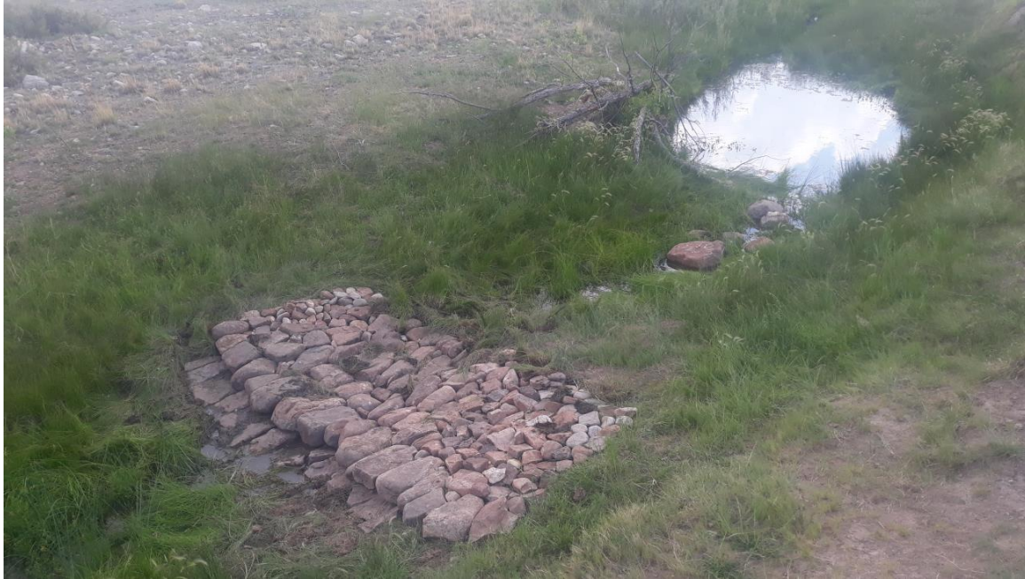
Figure 2. ORD structure and the wetland riparian vegetation surrounding the structure on Wolf Creek.
