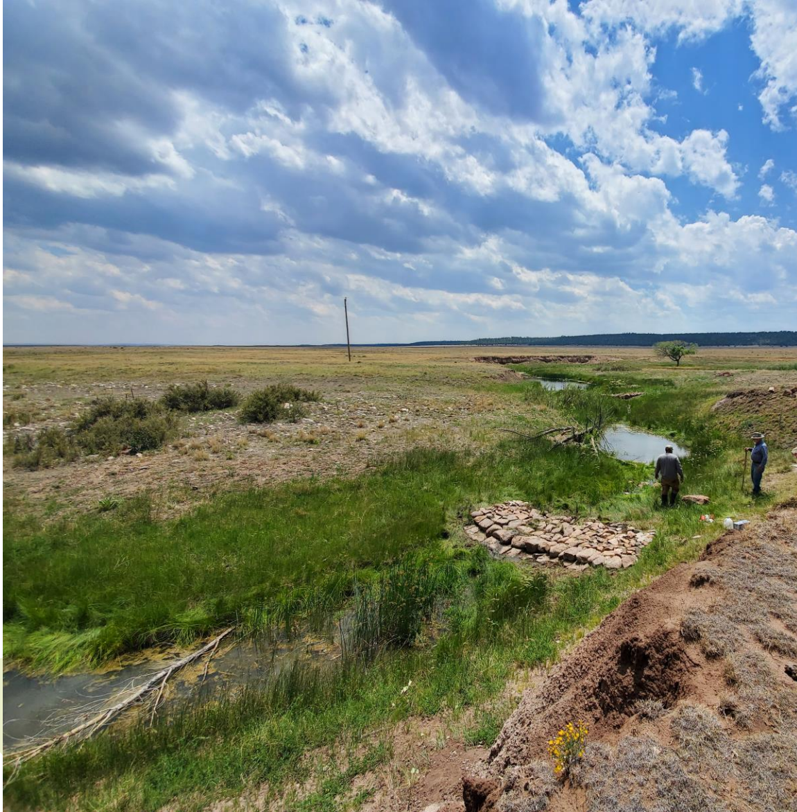
Figure 4. Bill Zeedyk directing the construction of an ORD structure.
