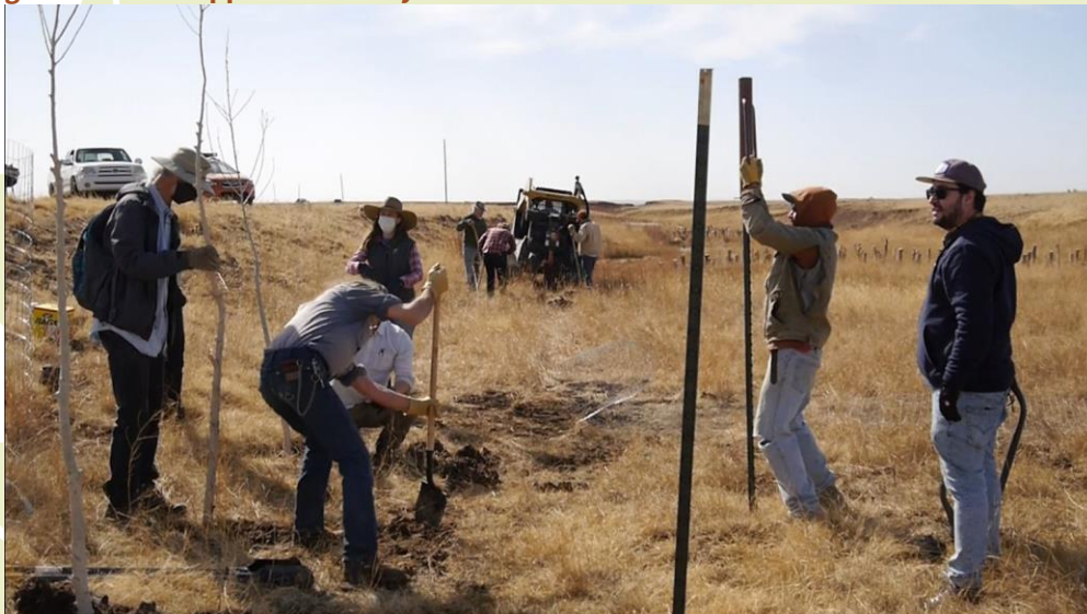
Figure 20. Volunteers from New Mexico Highlands University, helping construct small exclosure fences to promote successful regeneration of plated woody and herbaceous riparian species.
