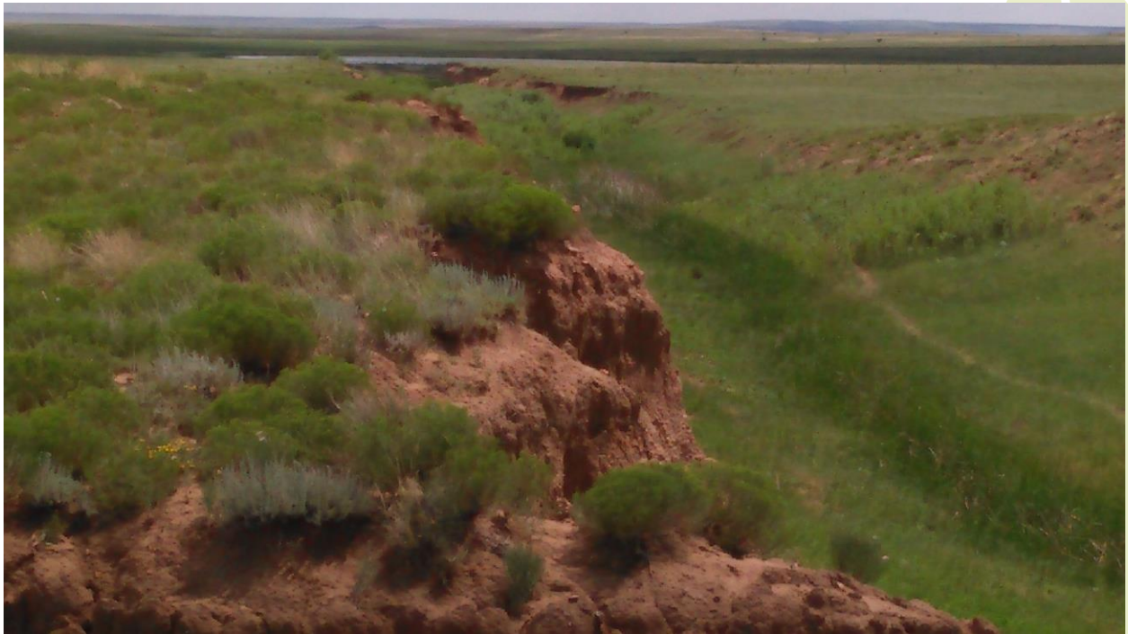
Figure 22. Wheeler Lake full of water in the background of the constructed inlet channel.
