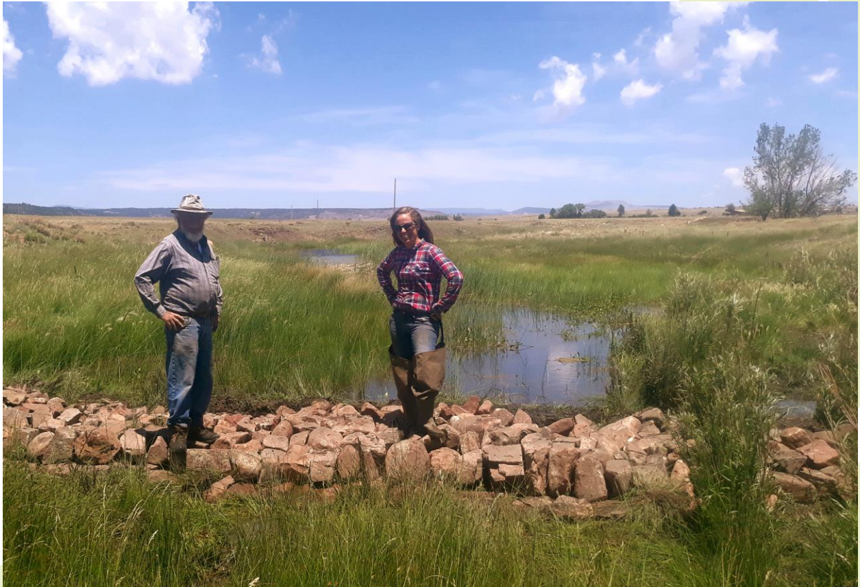
Figure 6. Bill Zeedyk and Amina Sena on the first constructed ORD, as part of an early training workshop.
