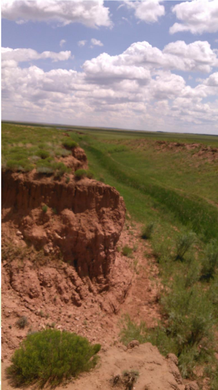
Figure 21. Constructed inlet to Wheeler Lake that diverts all Wolf Creek flows in this straight channel.
