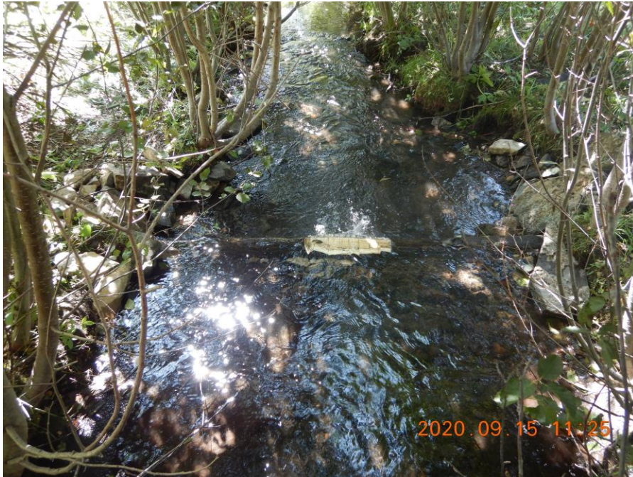
Man-made log dam repairs - LD 12 looking downstream after log notching.
