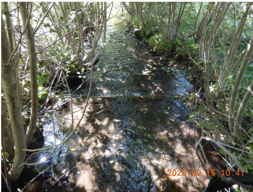
Man-made log dam repairs - LD 12 looking downstream before log notching.
